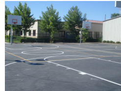
Resurfaced outdoor basketball court
