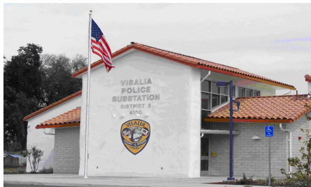
District 2 Police Substation
