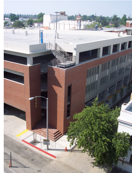
New Parking Structure
