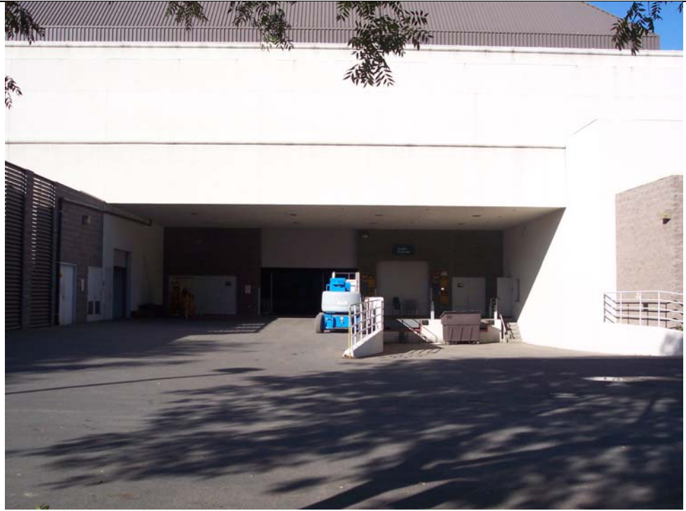
Picture 6-5 Loading Area
