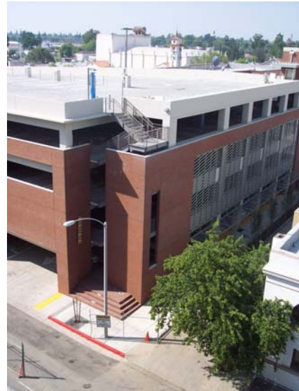
New Parking Structure
