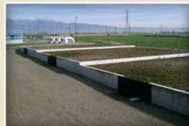
Volatile Organic Carbon Off-Gas Adsorption Units
