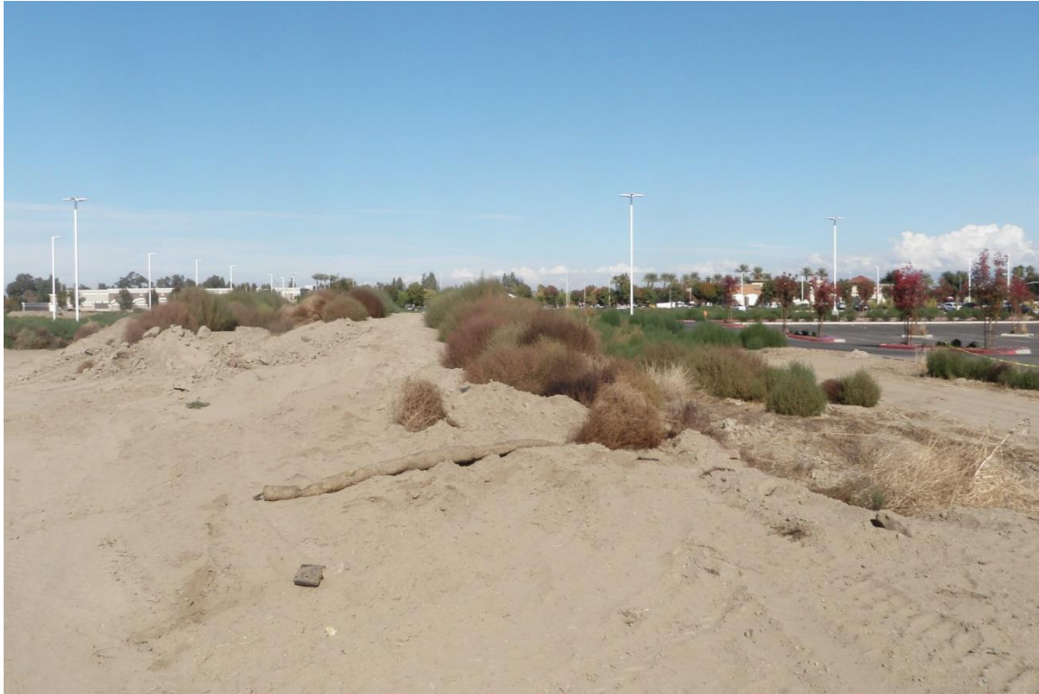
Figure 5 Overview of 6' stockpile of fill soils at the southwest corner of the project area. North
