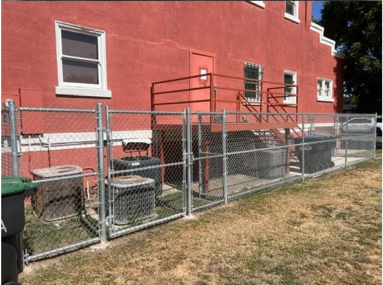
HPAC Item No. 2024-07 – 533 N. Locust St. – New Fence
