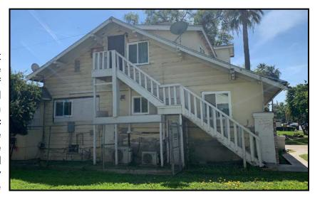
compatible with the stairway on the north side of the building. As such, Condition No. 1.c is recommended requiring that all stairs to be repaired shall be compatible with the existing staircase on the northern building exterior.
