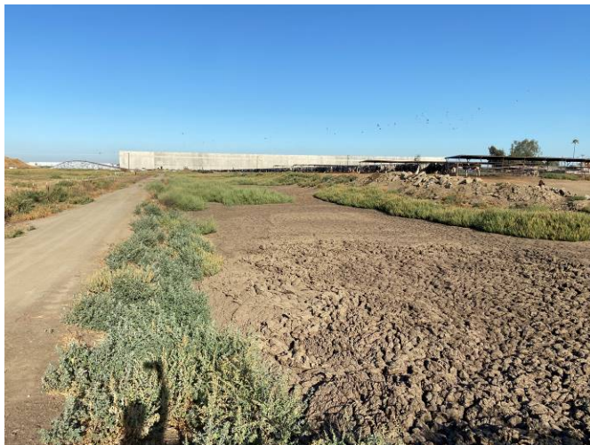
12. One of three effluent ponds.
