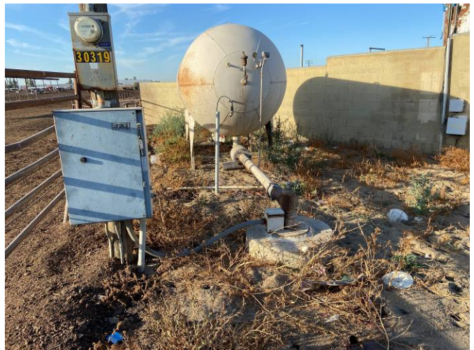
4. Water well at east side of milking barn.
