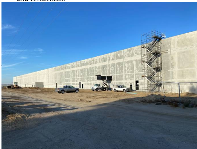
18. West adjoining under construction distribution warehouse.
