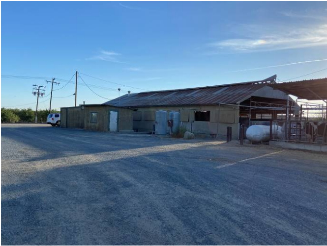
1. View of west side of on-site milking barn.
