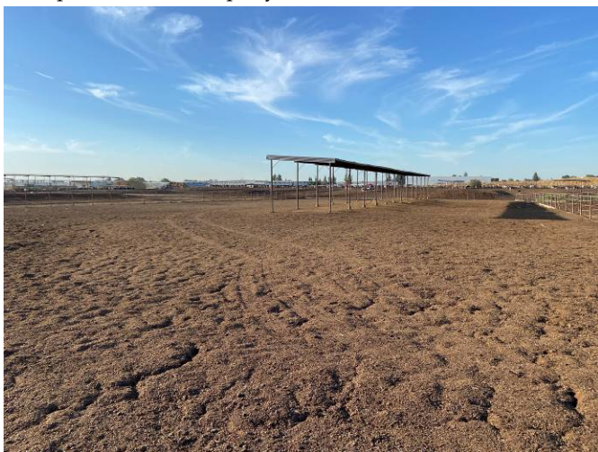
9. Corrals and shade structures.
