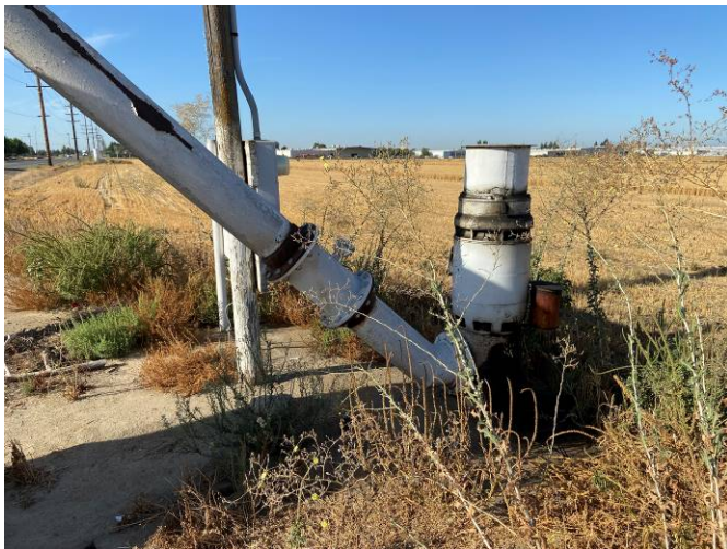
5. Irrigation well near east boundary of the Property.
