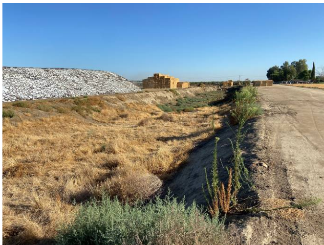
14. Eastern area of the final stage effluent pond.
