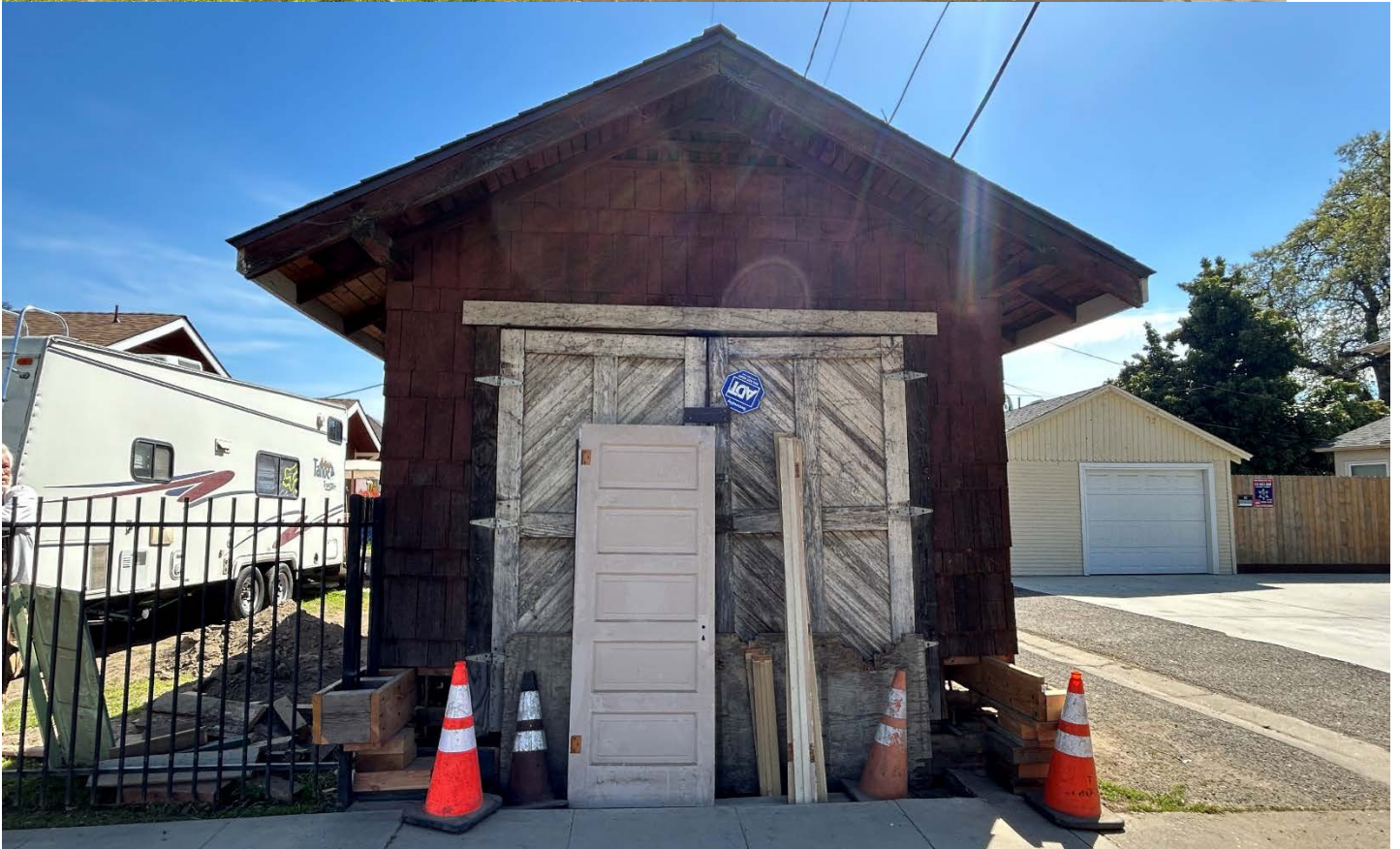
HPAC Item No. 2024-04 – Window and Garage Door Change Out
