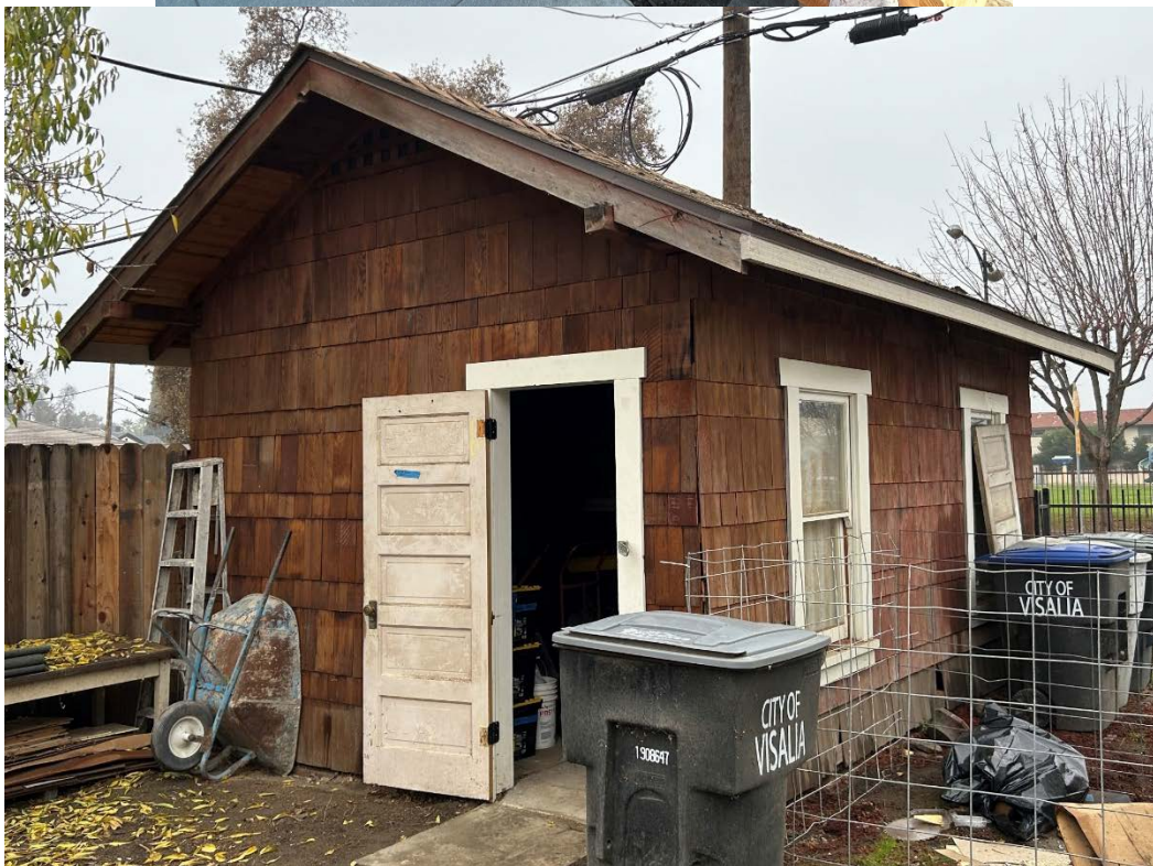
HPAC Item No. 2024-04 – Window and Garage Door Change Out
