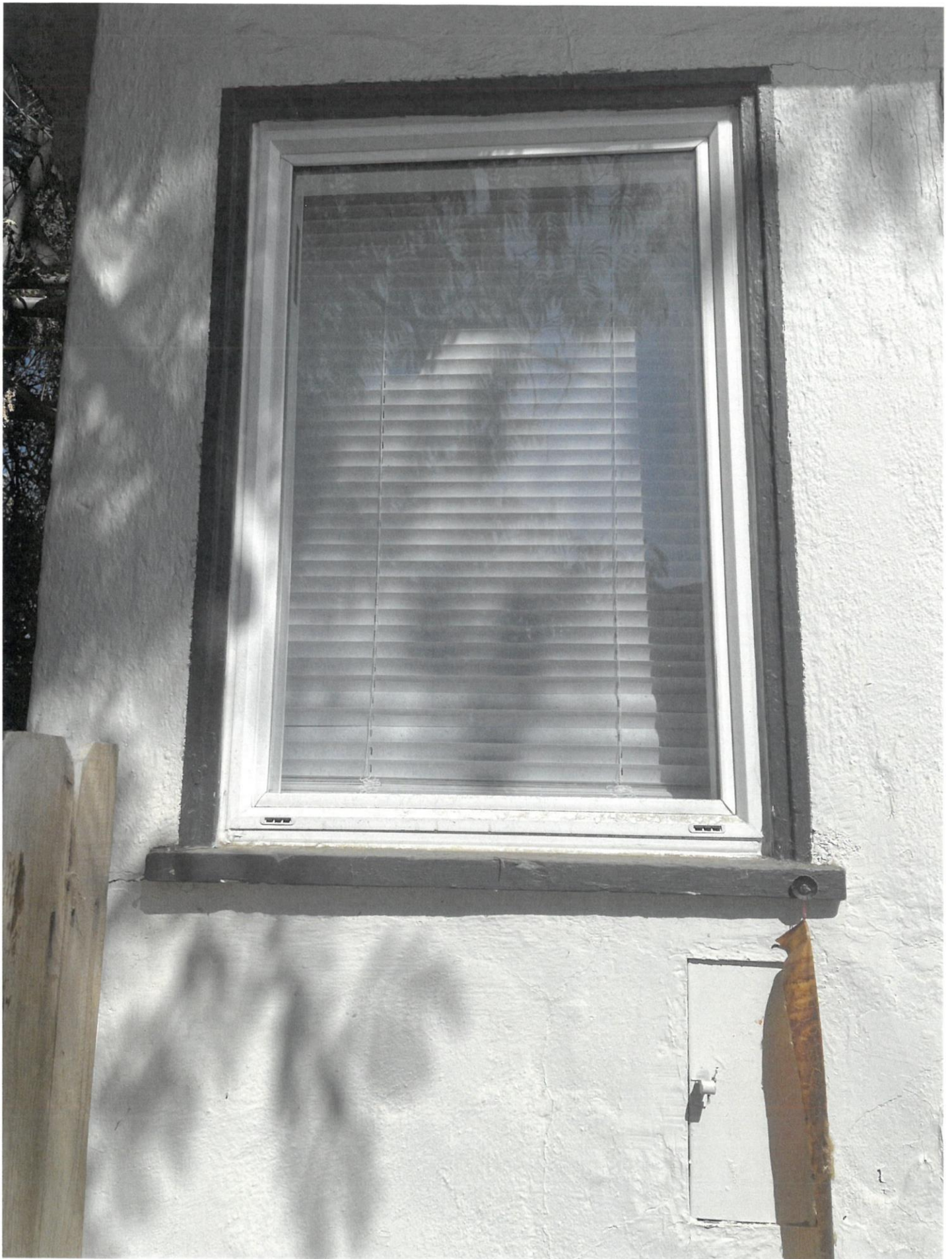
HPAC Item No. 2023-25 – 821 S. Court – Window Change Out
