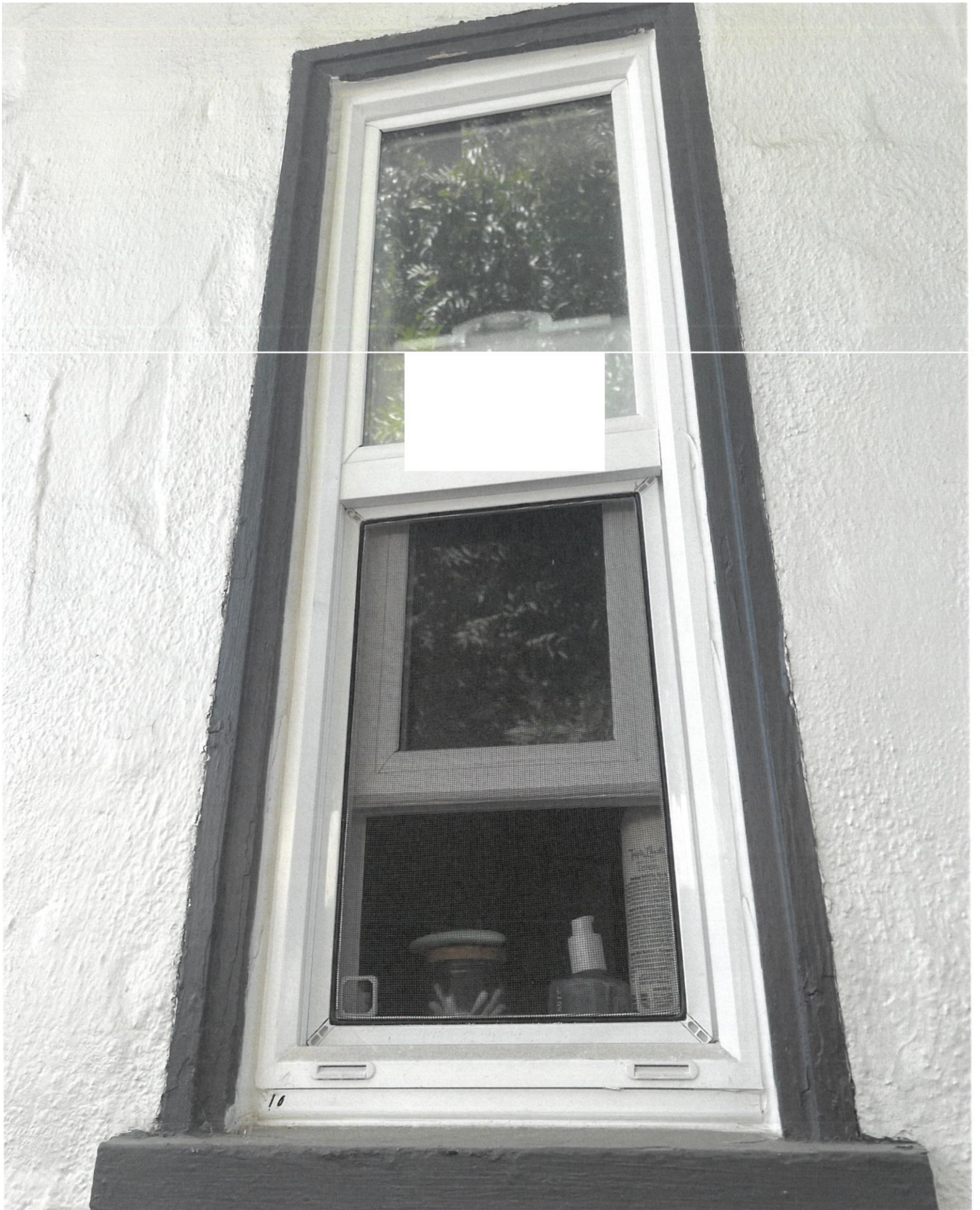
HPAC Item No. 2023-25 – 821 S. Court – Window Change Out
