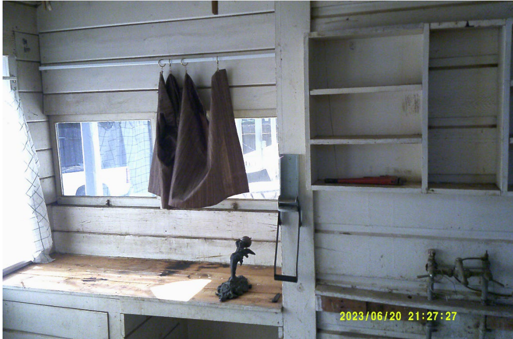
EXISTING LAUNDRY/SEWING SOUTH WALL
