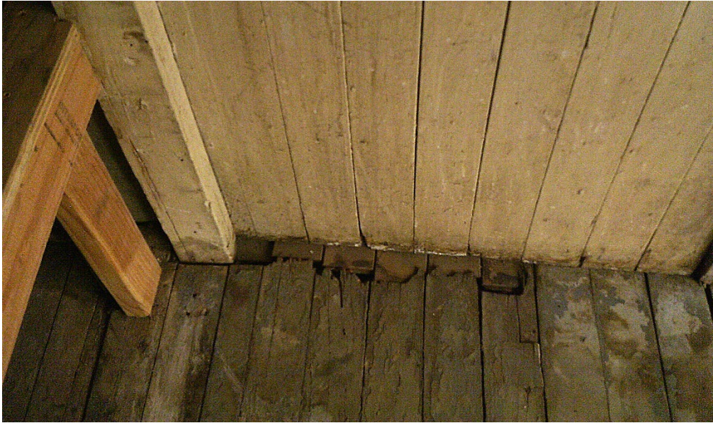
EXISTING LAUNDRY/SEWING NORTH WALL
