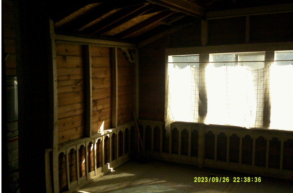
EXISTING LAUNDRY/SEWING NORTH-EAST WALL
