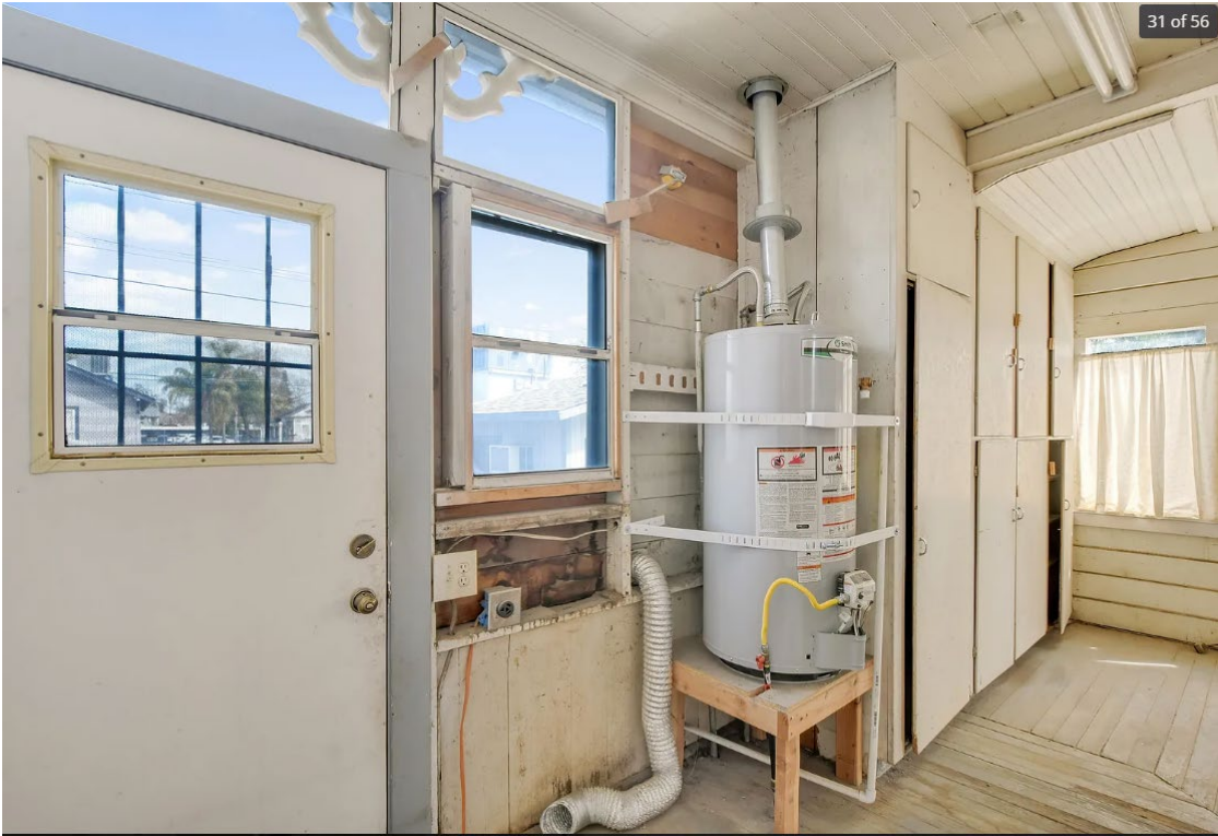
EXISTING LAUNDRY/SEWING NORTH WALL
