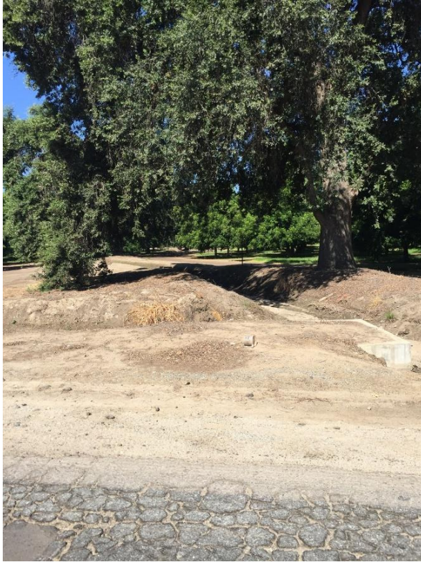
Figure 3-7. Road 152 at Oaks Ditch
