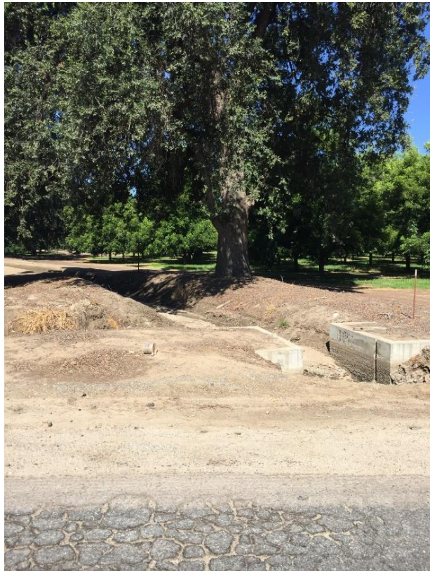
Figure 3-6. Road 152 at Oaks Ditch
