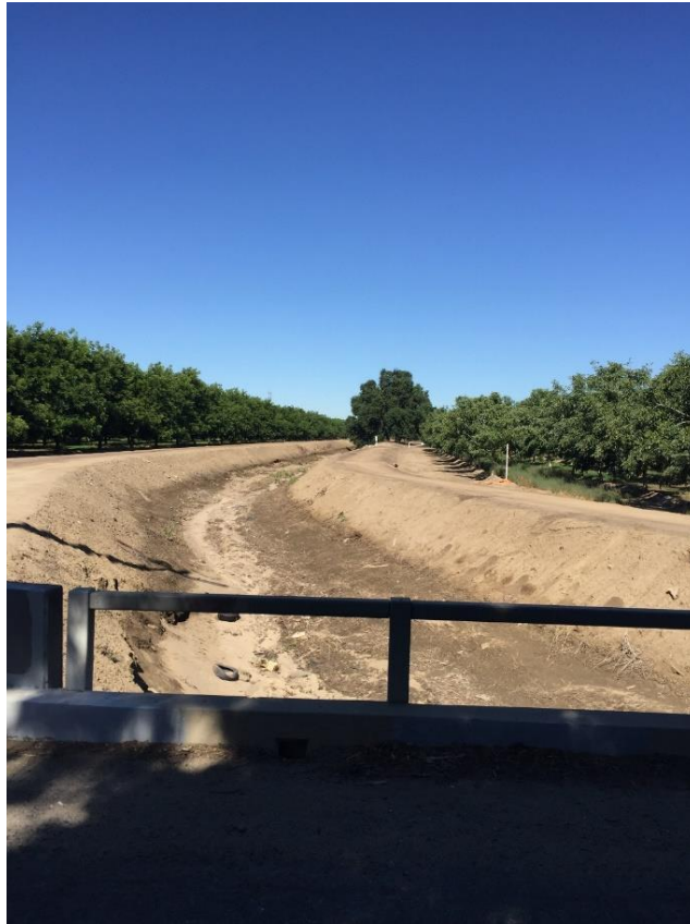
Figure 3-9. Road 152 at Mill Creek
