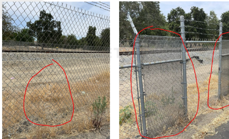
Multiple cuts and secondary repairs/reinforcements are constantly required
