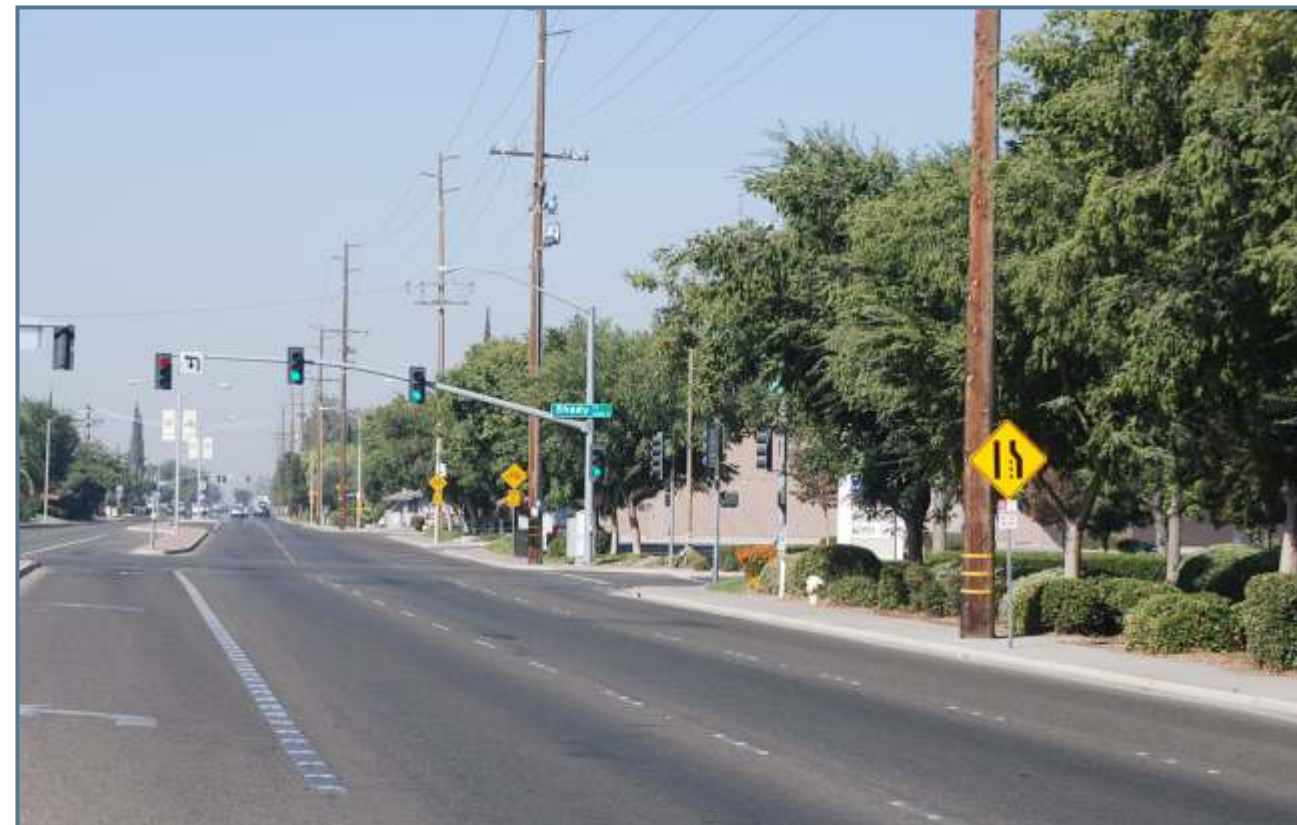
EXHIBIT 8 CALDWELL AVE. / WESTBOUND
