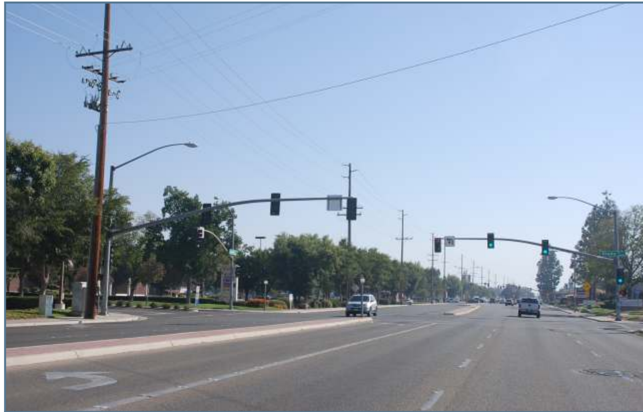
EXHIBIT 9 CALDWELL AVE. / EASTBOUND
