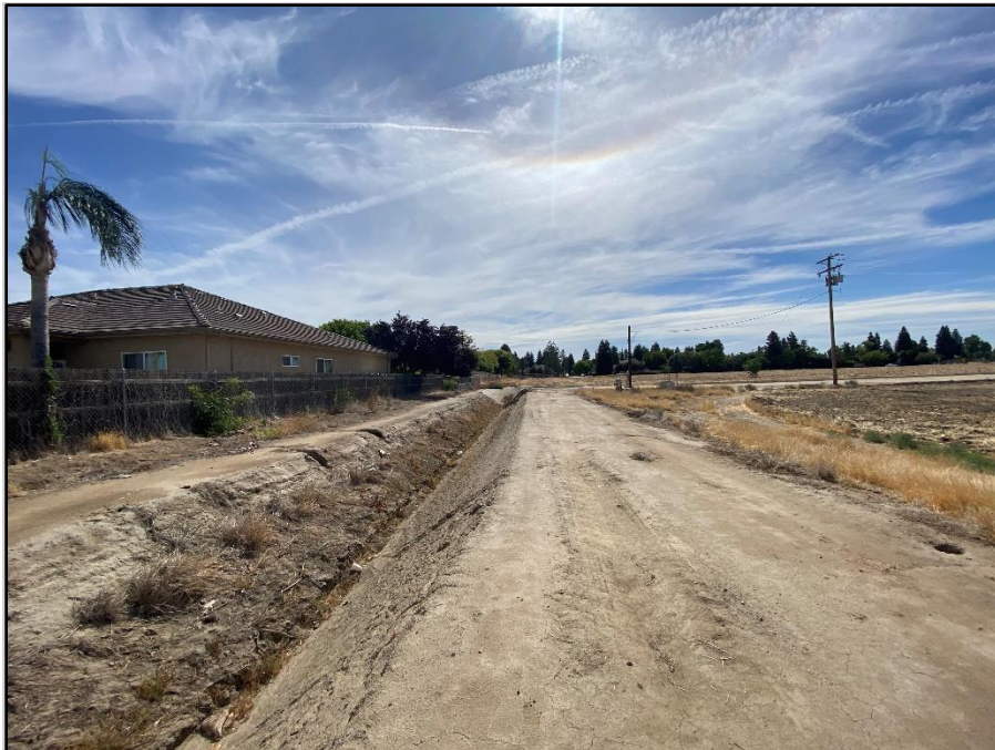
Figure 4-8 South Fork Persian Ditch on the Project site, facing east.
