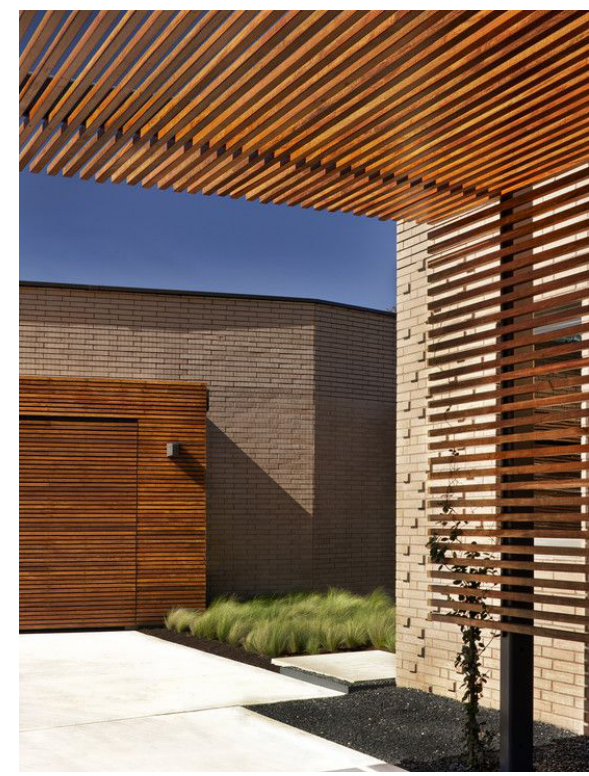
WRAPPING WOOD SHADE STRUCTURE
