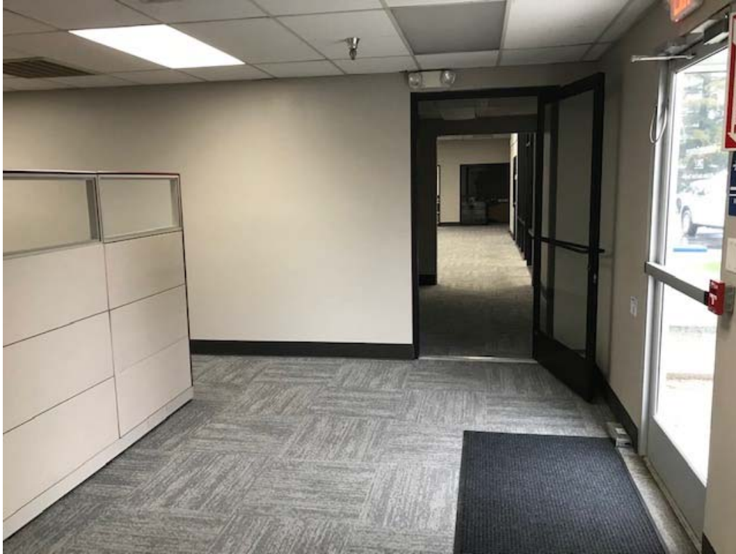
Entrance door on right, cubicle on left, will have receptionist counter installed back on.
