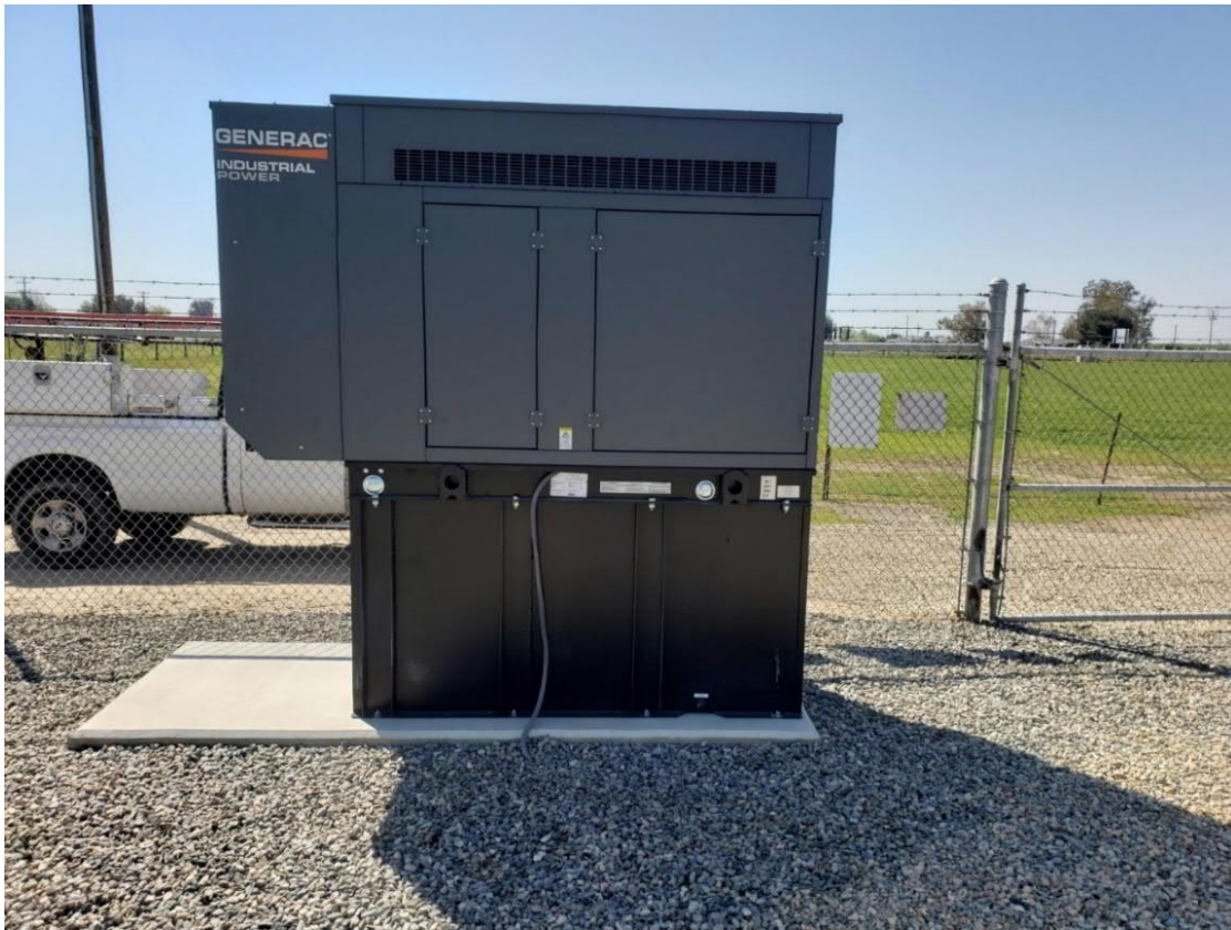
Above: View of typical 25kW Generac diesel generator.
