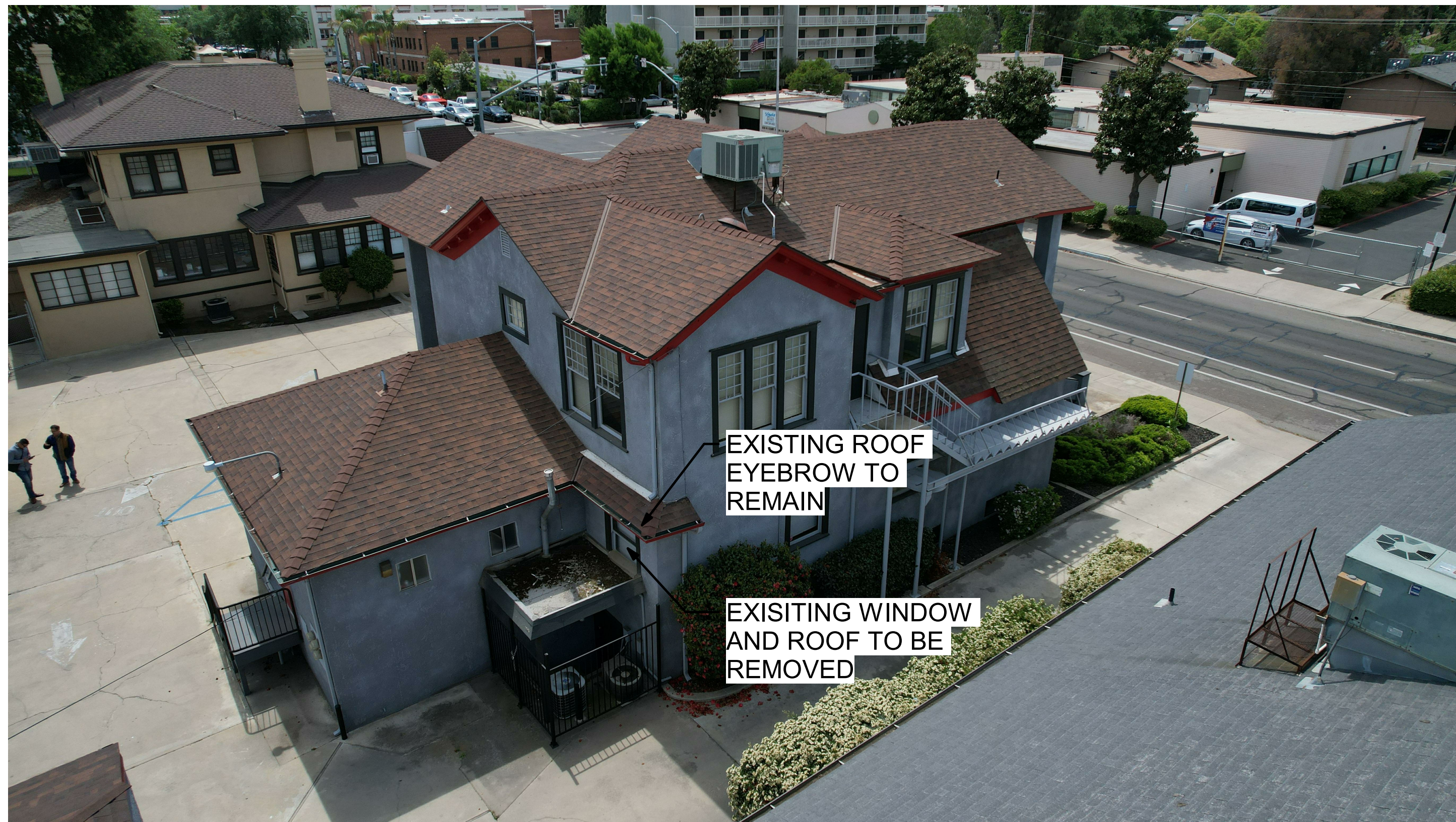
EXISTING NORTH ELEVATION
