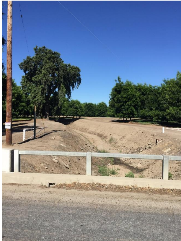
Figure 3-5. Road 152 at Packwood Creek
