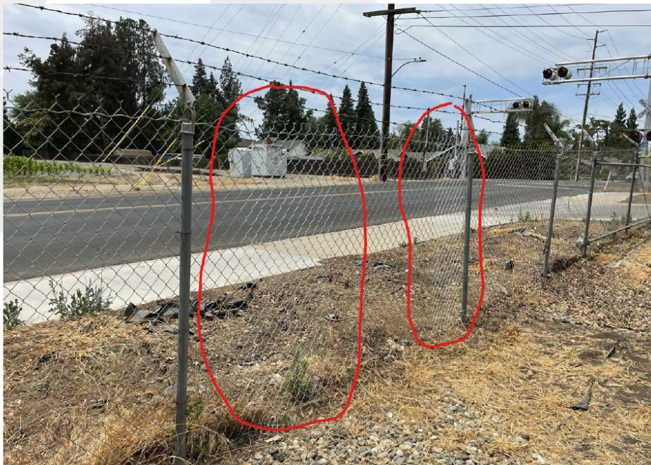
Fence repairs are a financial hardship due to ongoing criminal breach into the property.
