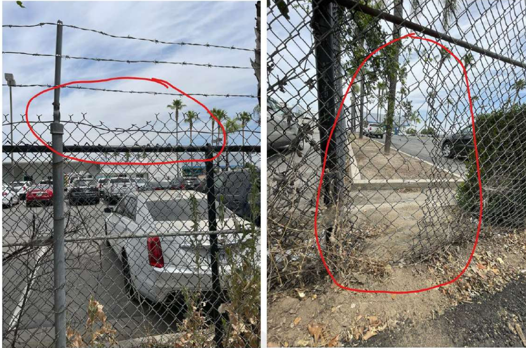
Neighboring property being used by criminals as a gateway entry/exit point
