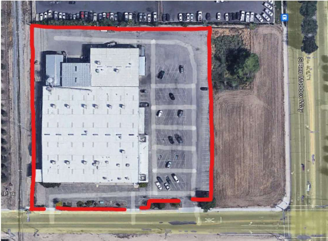
(Multiple areas of the property boundary are breached through the existing fence)
