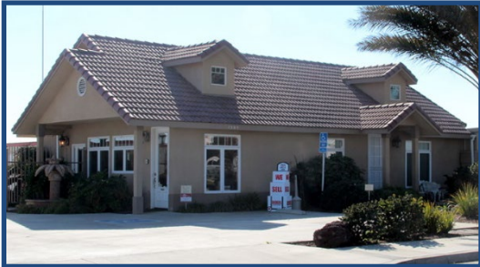
Before Main Office Building
