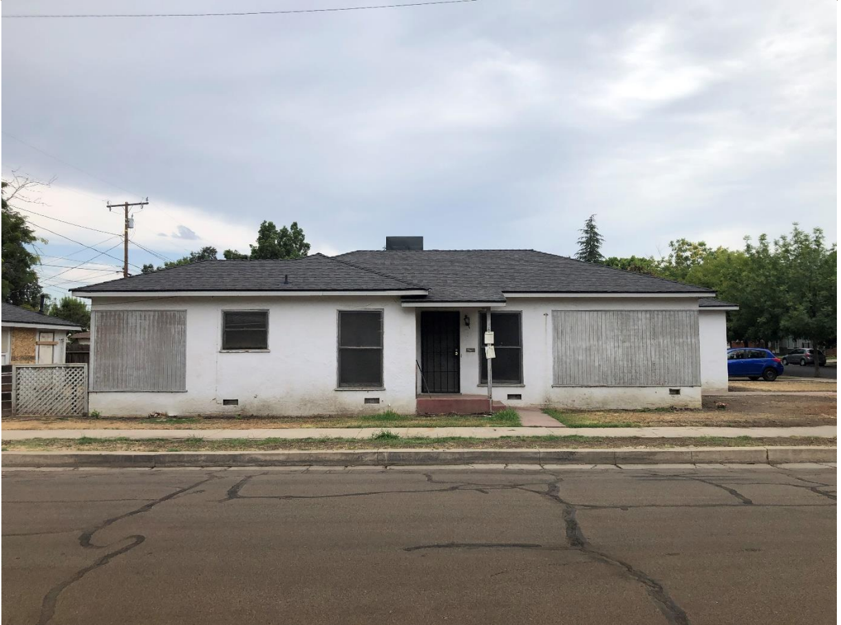
HPAC Item No. 2022-15 – Exterior Alterations
