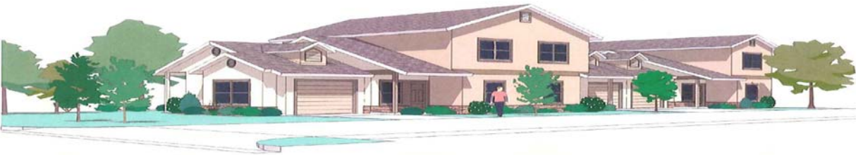
Below: Elevation of existing eleven (11) units after rehabilitation
