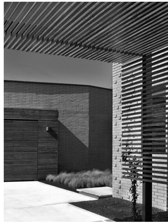
WRAPPING WOOD SHADE STRUCTURE
