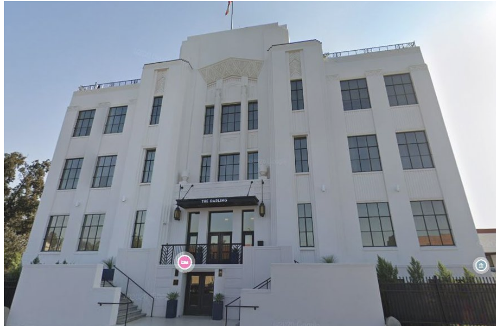
④ DARLING HOTEL - MAIN BUILDING
