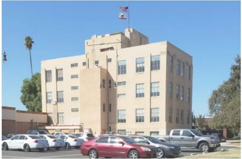
EXISTING REAR FACADE OF VISALIA COURTHOUSE
