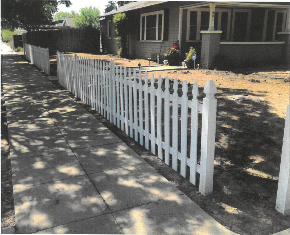
HPAC Item No. 2021-04 – New Fence
