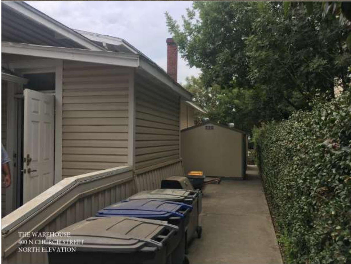
HPAC 2020-07 - 400 N. Church Street - The Warehouse
