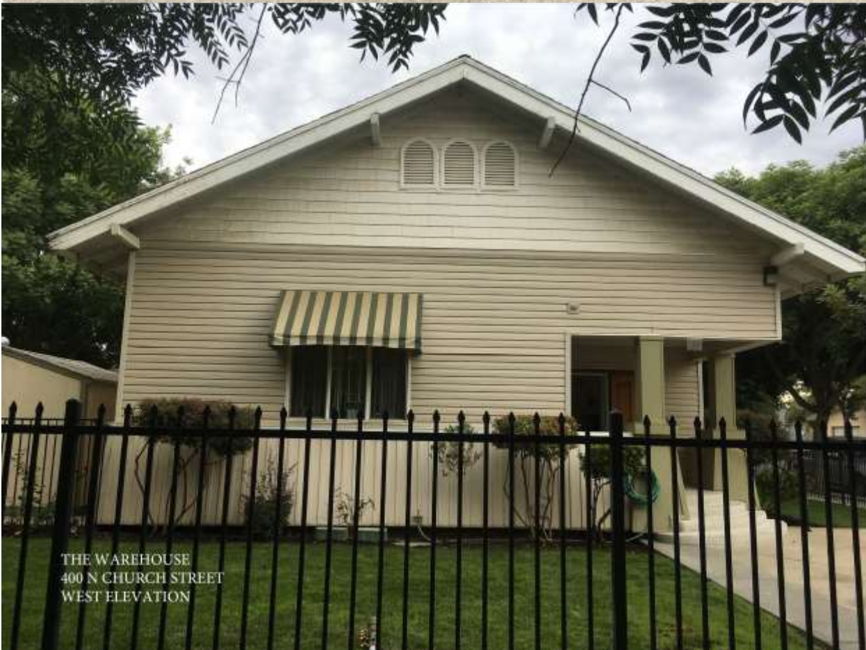
HPAC 2020-07 - 400 N. Church Street - The Warehouse
