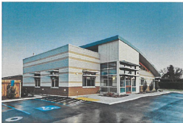
EXISTING LAB BUILDING: ENTRANCE
