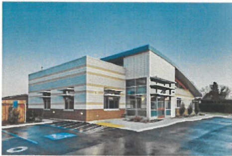
EXISTING LAB BUILDING: ENTRANCE
