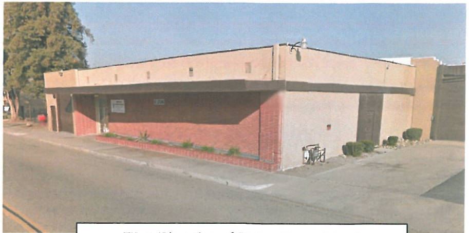
West Elevation of 700 S. Bridge Street
