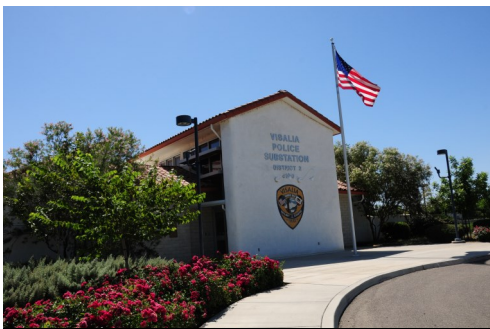
District 2 Substation located at 4100 South County Center.
