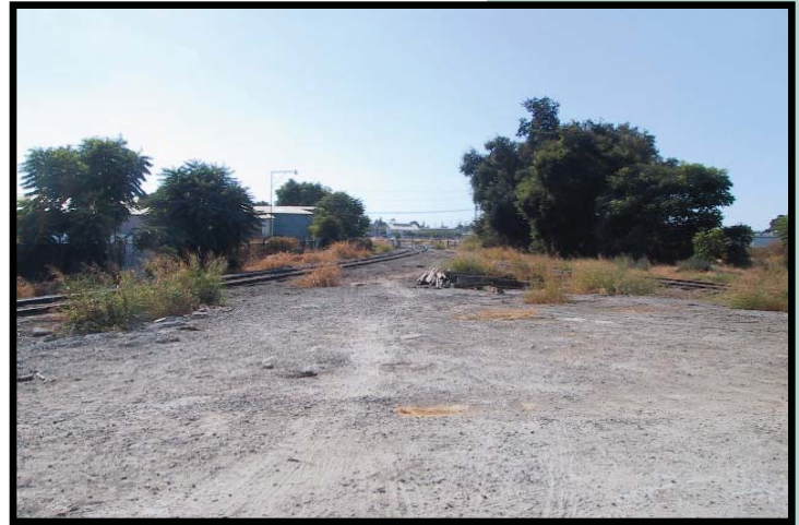
View north as tracks branch bordering future storm basin open space area (See Chapter 11).
