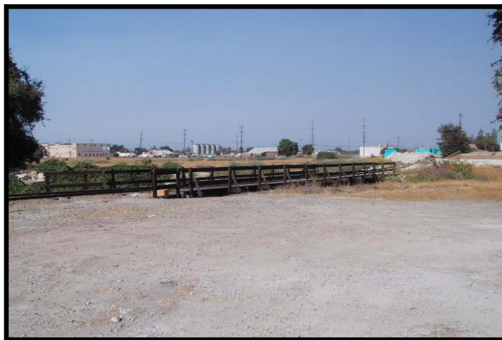
View northwest of existing railroad trestle over Mill Creek.
