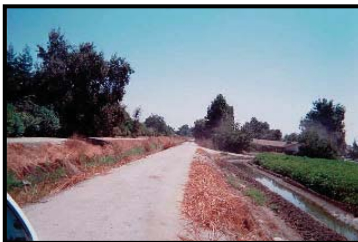
View west along Mill Creek near Manzanita Street.
