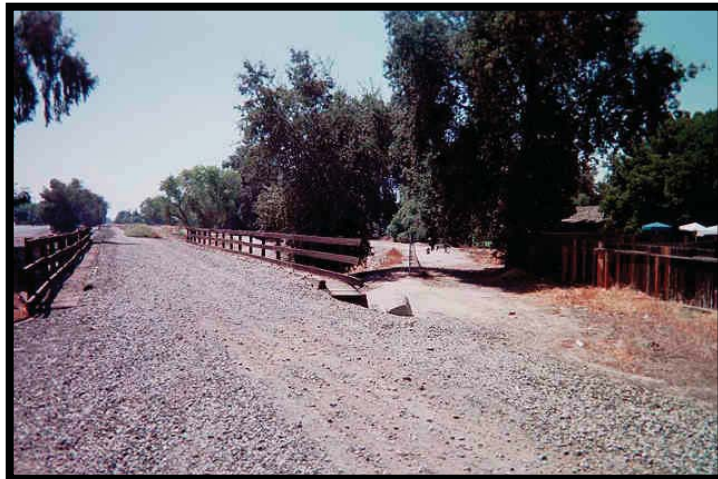
View due south from old Santa Fe trestle crossing Packwood Creek.
