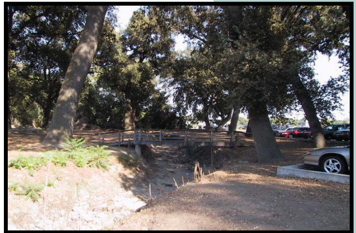
View west of bridge crossing Mill Creek under the Oak preserve canopy.
