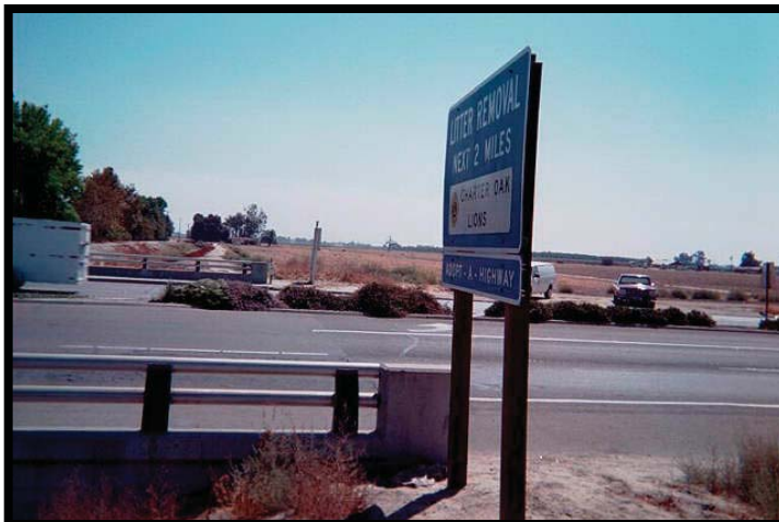
View east to Packwood creek culvert crossing at Mooney Blvd.. at the future signalized Cameron Ave. intersection
