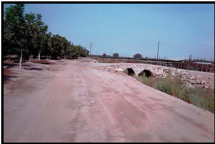
View northeast to existing Culvert Crossing, potential rest area and viewing.
