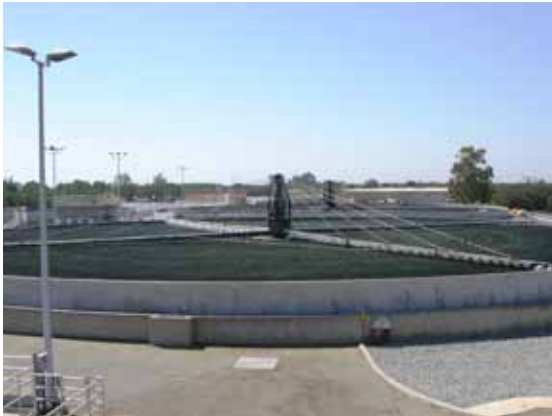
Surface water treatment and delivery may become necessary over time as ground water depths increase. (Top)
