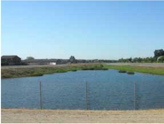
Visalia's storm drainage system relies on detention basins and several retention basins to slow and divert storm water for larger storms.
