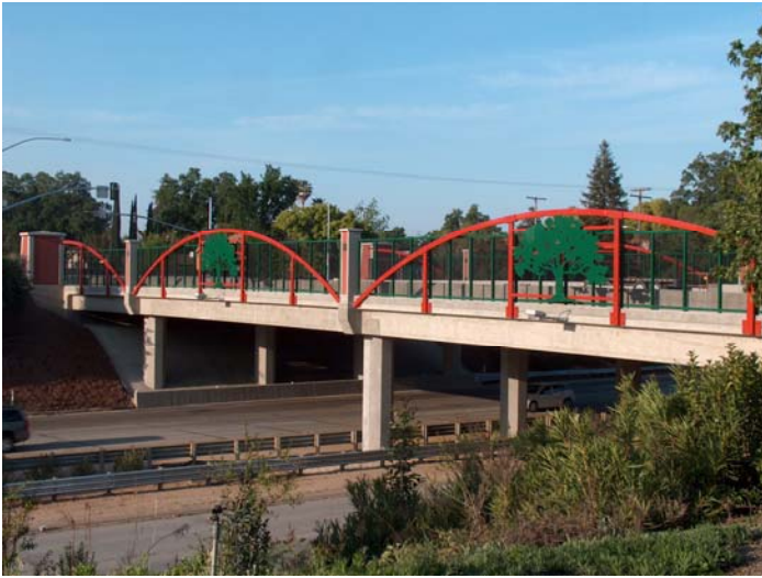
Santa Fe Bridge
