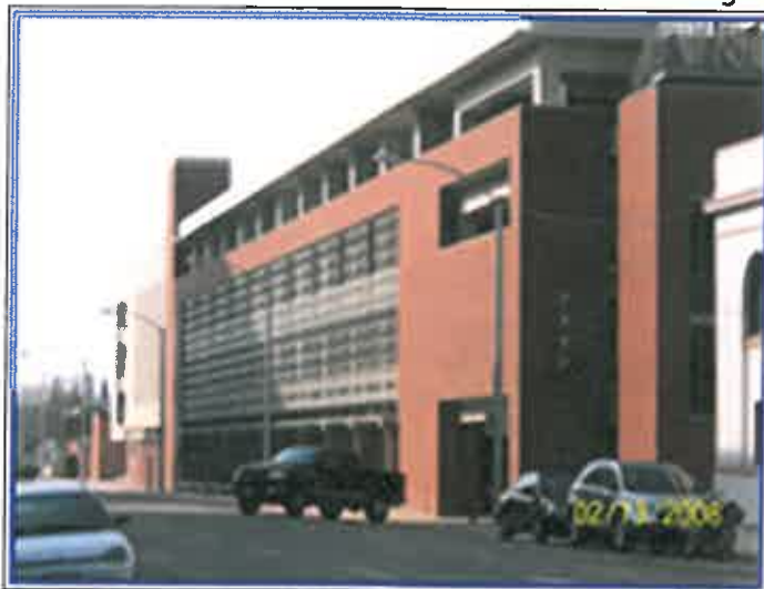
Image 7: West Acequia Parking Structure
