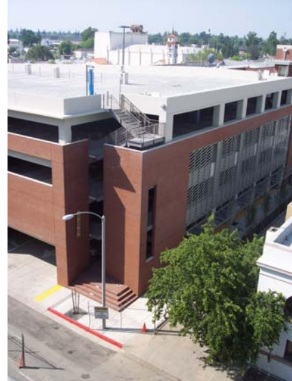
New Parking Structure
