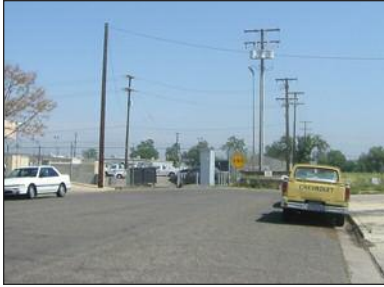
Above: School Street extension area view from west
