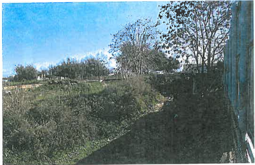
View of existing conditions of Mill Creek between Tipton and Burke Streets, an 8-ft fence borders the channelized waterway
