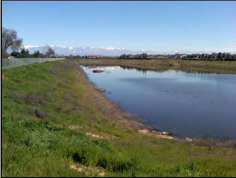
Shannon Ranch Basin Demaree & Shannon Parkway February 28, 2011
