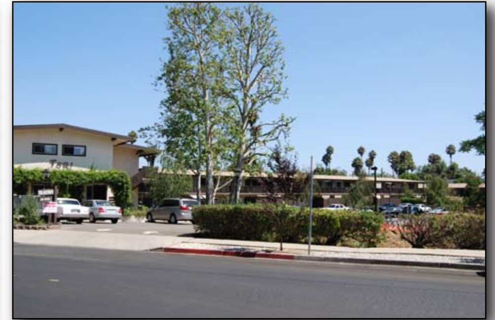
Location 6 - Existing San Remo Drive at T&C Apartments
