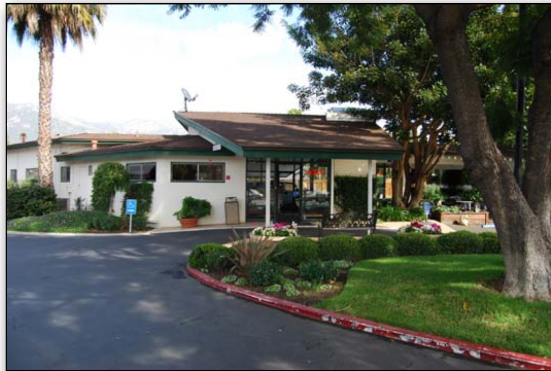
Existing Hotel Office
