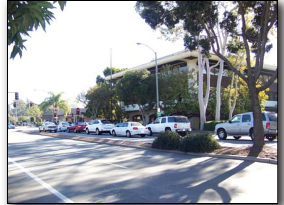
Location 9 - Looking Southeast State Street West of Project Site
