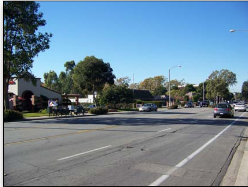
Location 12 - Looking Southwest State Street at San Roque Creek
